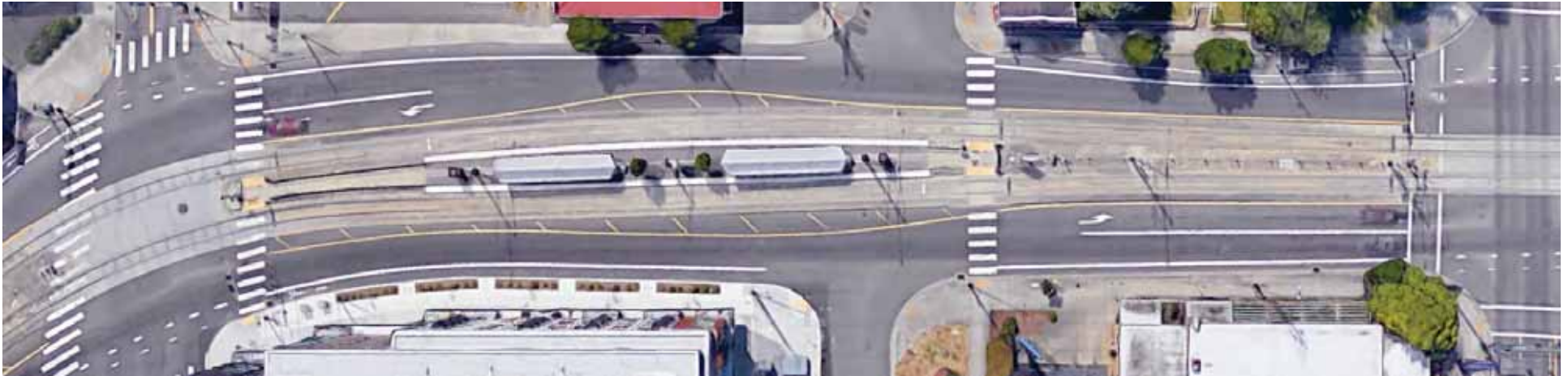
On-street parking was removed at the N Prescott St. MAX station to maintain a continuous bike lane and provide space for a left-turn lane. Image from Google Earth
