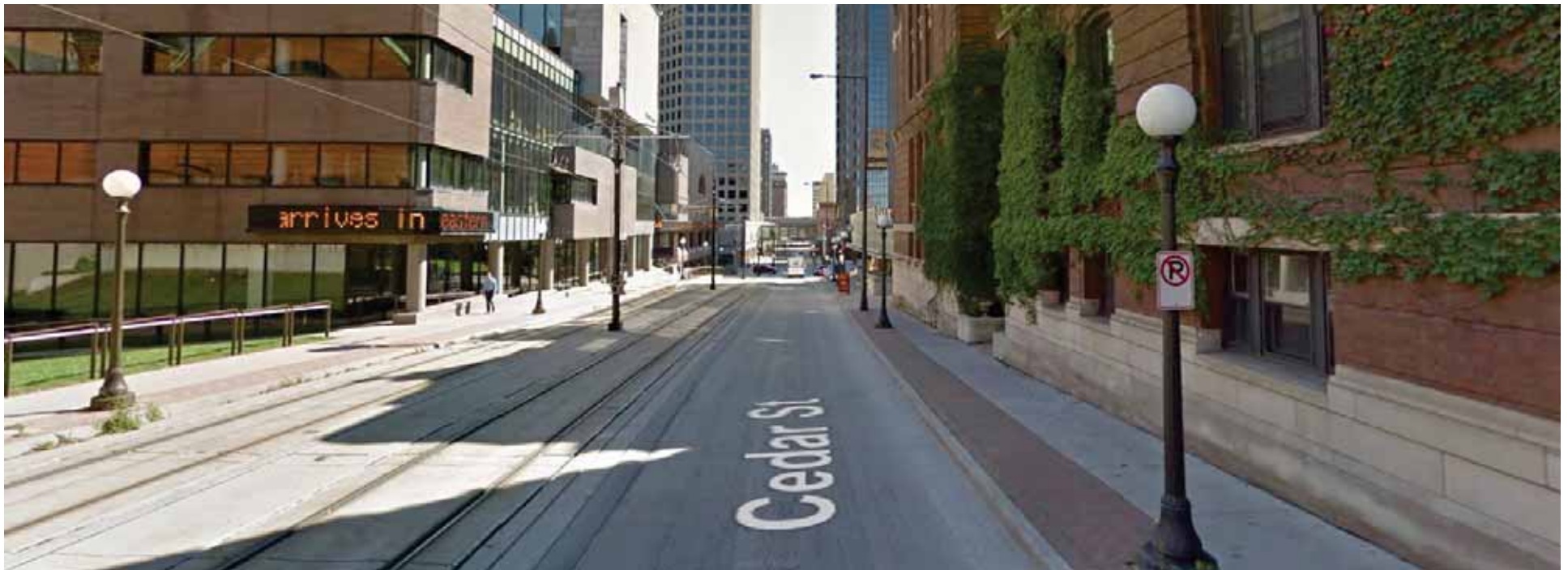
Cedar Street downtown St. Paul is shown in 2015 following construction of the Metro Green Line. This street hosts two-way light rail as well as a single southbound traffic lane. Consolidating light rail operations on this street avoided impacts to adjacent streets in downtown St. Paul.
