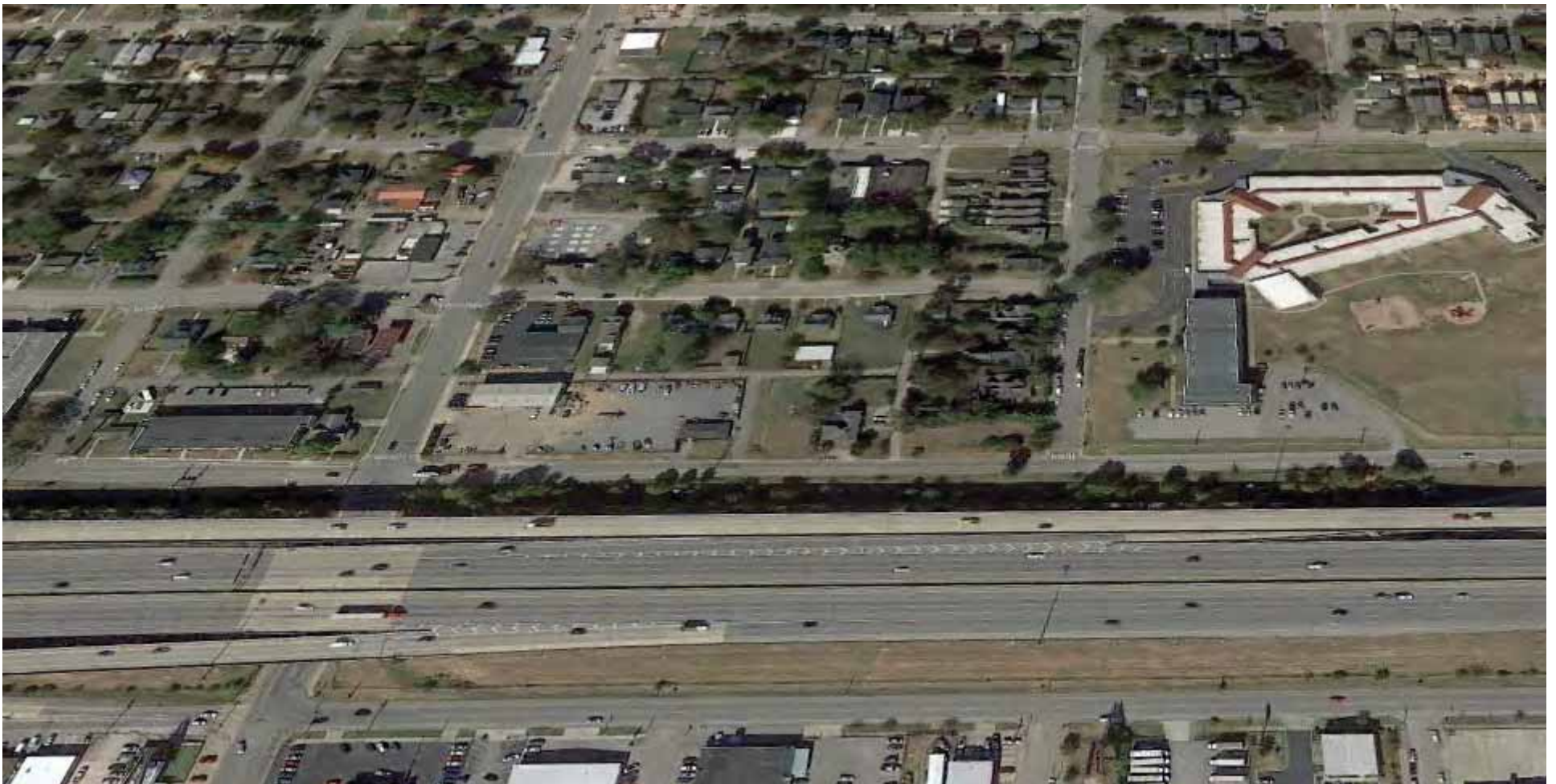
The neighborhoods North of I-40 can be connected to the high capacity transit along 51st Avenue and 46th Avenue.
