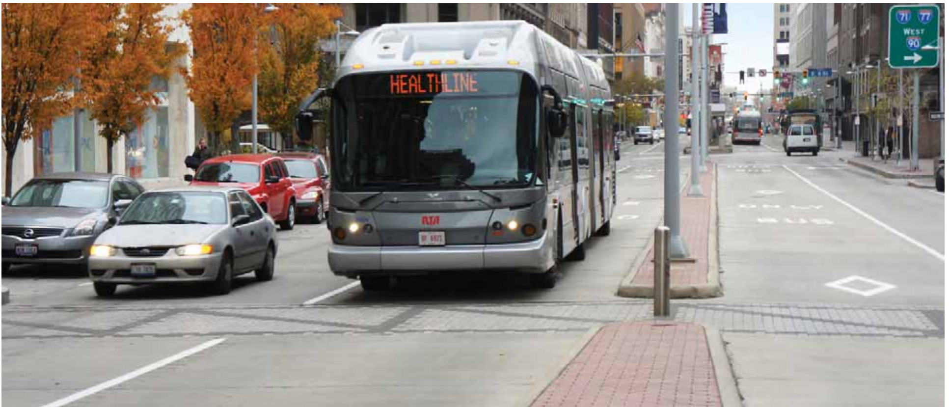
Construction of the Healthline BRT in Cleveland removed traffic lanes from Euclid Avenue but added bicycle lanes and widened sidewalks. Image from Nolan Levinson
