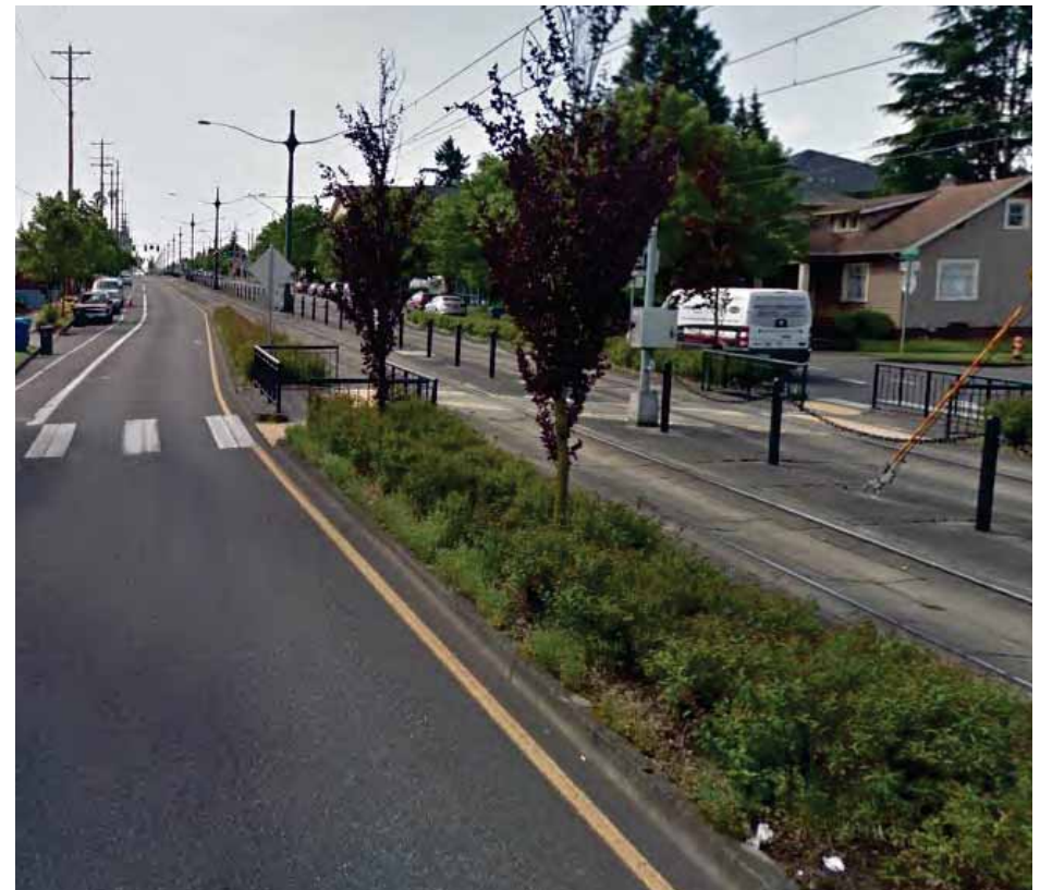
The MAX Yellow Line project provided high-quality pedestrian crossings of Interstate Avenue. Bicycle lanes were maintained at these crossings by eliminating on-street parking spaces.
