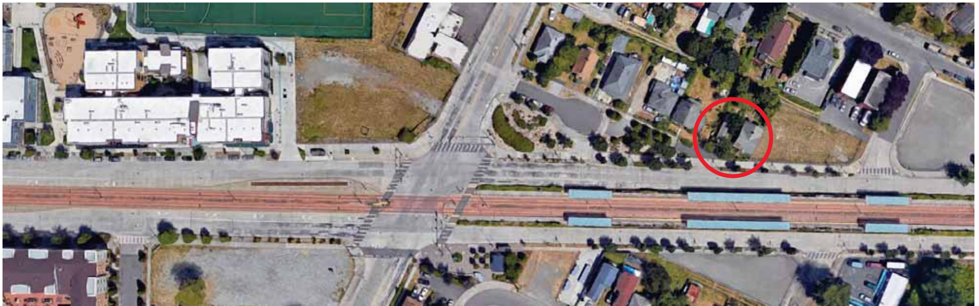
Construction of Central Link light rail in Seattle required widening the right-of-way along Martin Luther King Jr. Way by three feet or more. Widening was minimized to avoid private property impacts where possible; the house circled in red is now just a few feet from the sidewalk.
