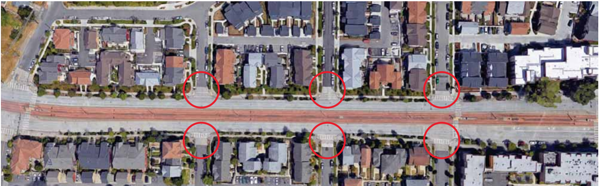
This segment of MLK Jr. Way shows where several intersections have been converted to right-in/right-out use only (circled in red). Restricting left turns throughout the corridor has allowed for high speed and reliability on Central Link’s street-running sections in Seattle.
