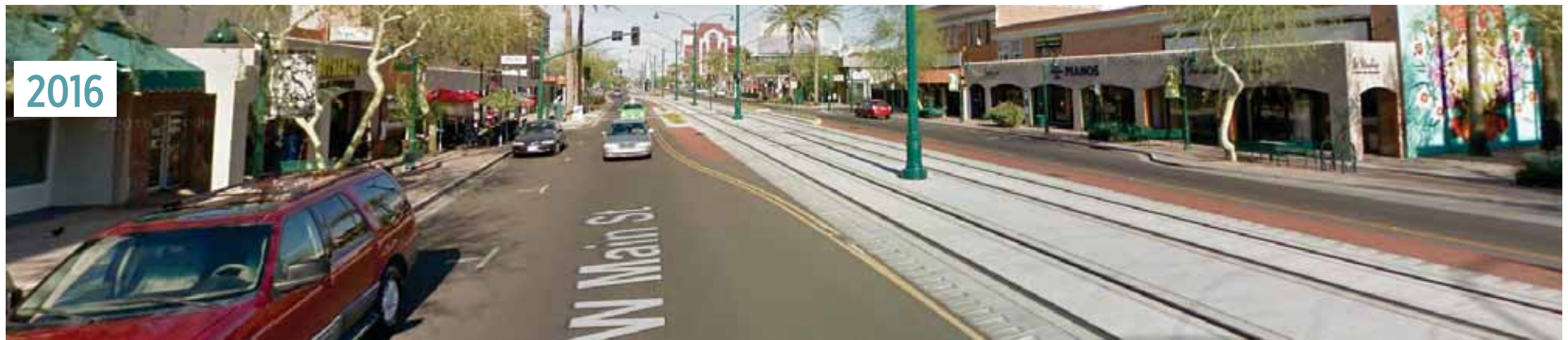
Main Street in downtown Mesa is shown in 2016 following construction of the Valley Metro Light Rail. Traffic lanes and bike lanes were eliminated to maintain on-street parking and wide sidewalks.
