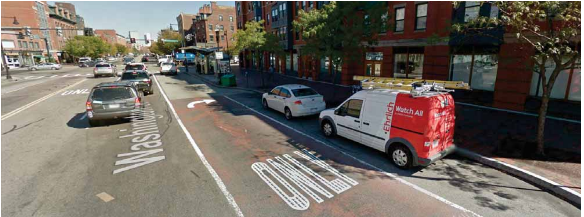
The Silver Line BRT corridor along Washington Street in Boston shares bus lanes and stations with right-turning traffic and cars accessing on-street parking. Shared use of these bus lanes has resulted in low speed and reliability compared to other high capacity transit systems.
