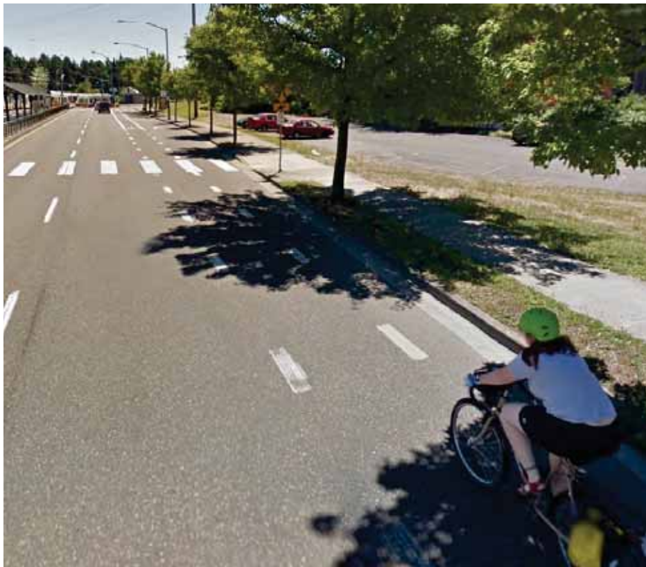
The MAX Yellow Line in Portland prioritized continuous bicycle lanes over general purpose travel lanes and on-street parking. For example, on-street parking was removed at constrained locations like this station platform at Prescott Street to provide room for a bike lane.
