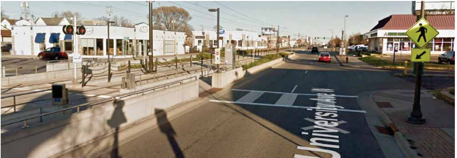
Most of University Avenue's on-street parking in St. Paul was removed to build the Metro Green Line. Hundreds of parking spaces were removed to make room for pedestrian crossings like the one shown here, prioritizing pedestrian access to light rail.
